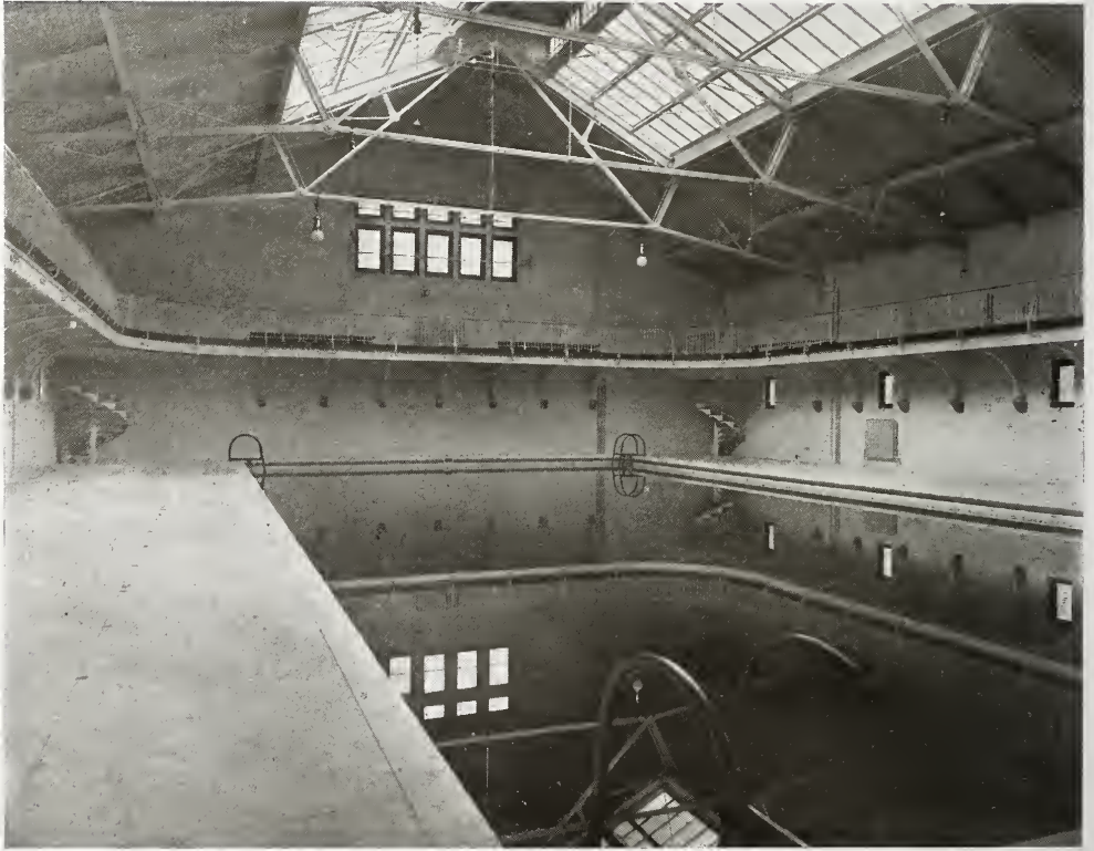
SWIMMING POOL—U. S. MILITARY ACADEMY, WEST POINT, N. Y. Cram, Goodhue & Ferguson, Architects, 1908.
